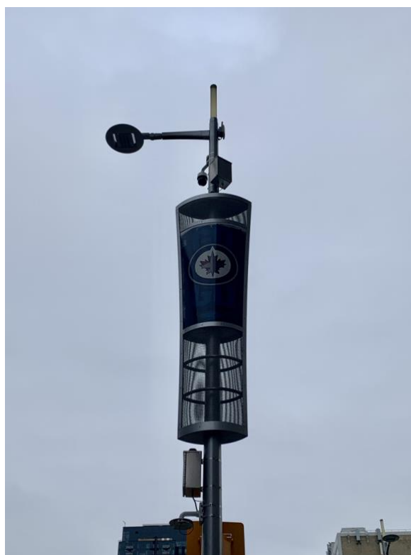
Image 4: CCTV Camera above Jets Logo Sign and broken/removed CCTV Camera below sign. Corner of Graham Avenue and Donald Street.
